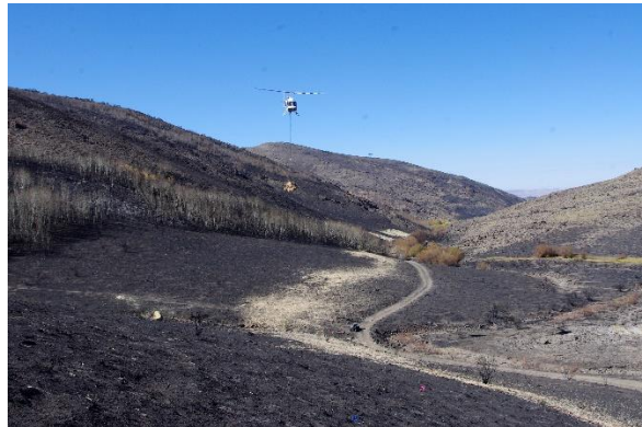
Figure 13. Helicopter application of WoodStraw ® to form sediment capture strips along seasonal creek on BLM Willow Fire. Multiple passes make the stripe wider at low points with higher expected flow.
