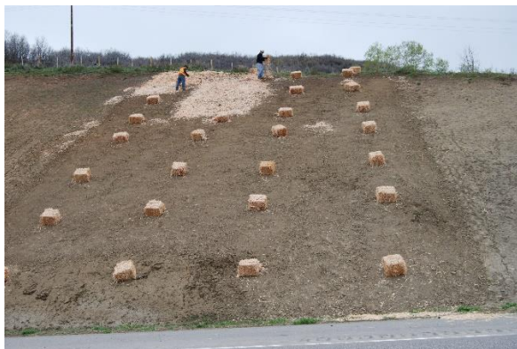
Figures 7. Hand application of wood-strand mulch at 70% soil cover on a 51% slope in Colorado in a CDOT test and follow-up two months later.
